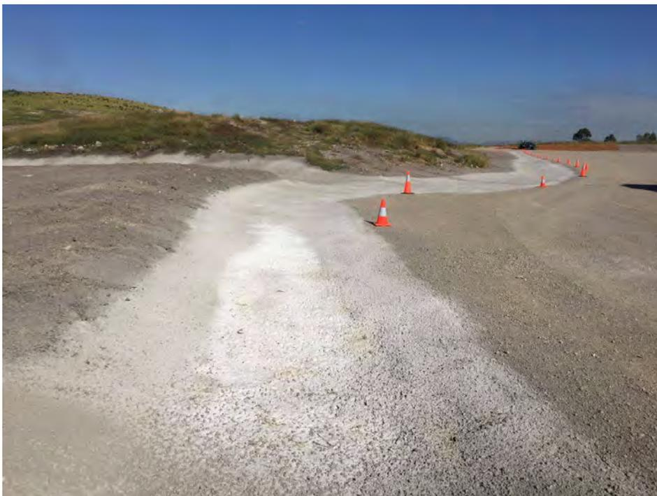
Photo 6 Looking along the composting pad southern perimeter surface drain, leading to the spillway
