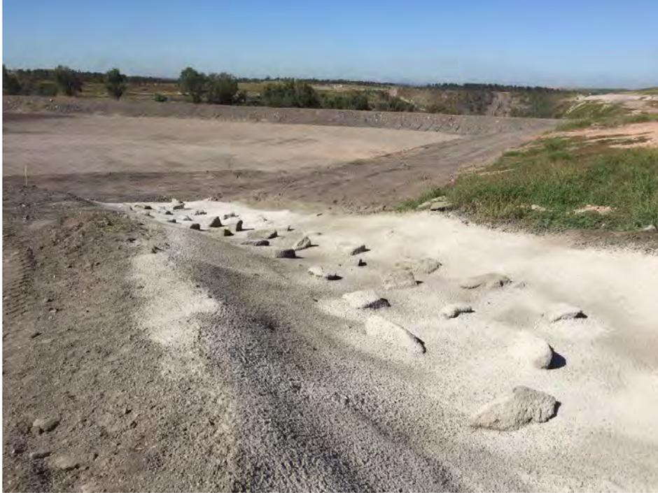
Photo 3 Looking down the shotcreted spillway channel
