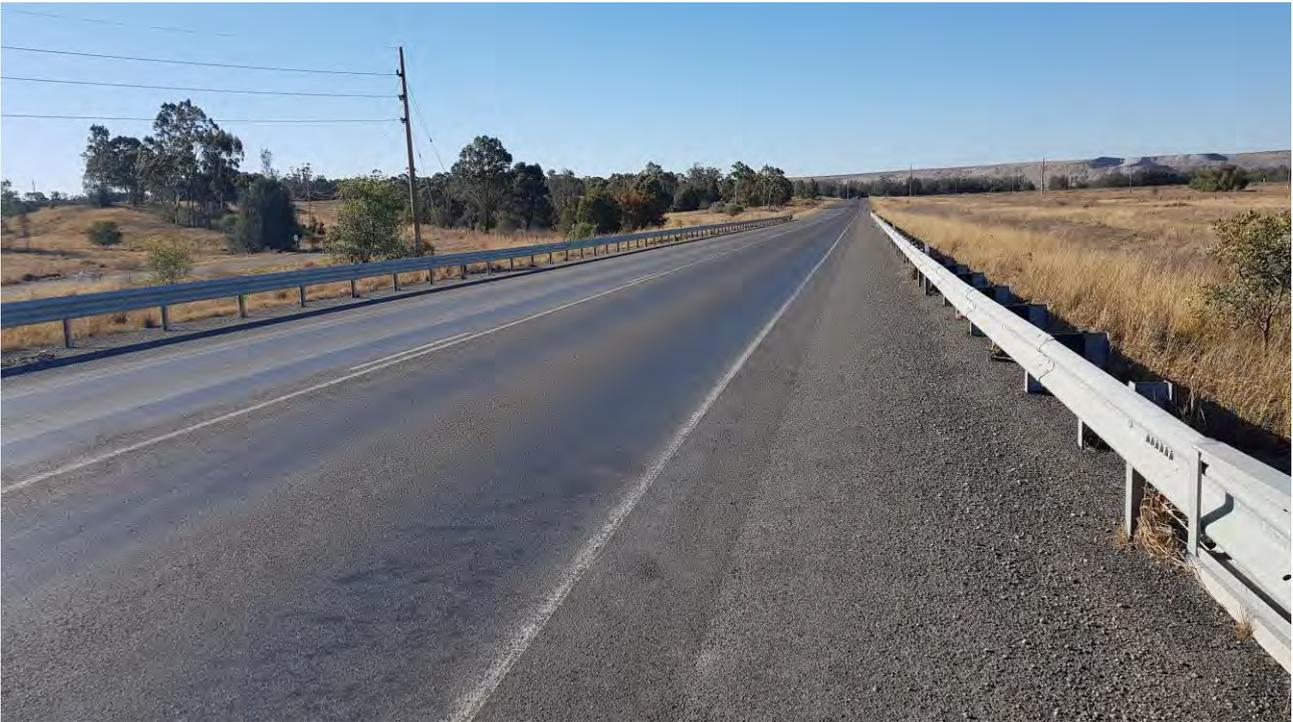
Figure 6 - Looking North-East, no defects in laneway, minor wear in shoulder
