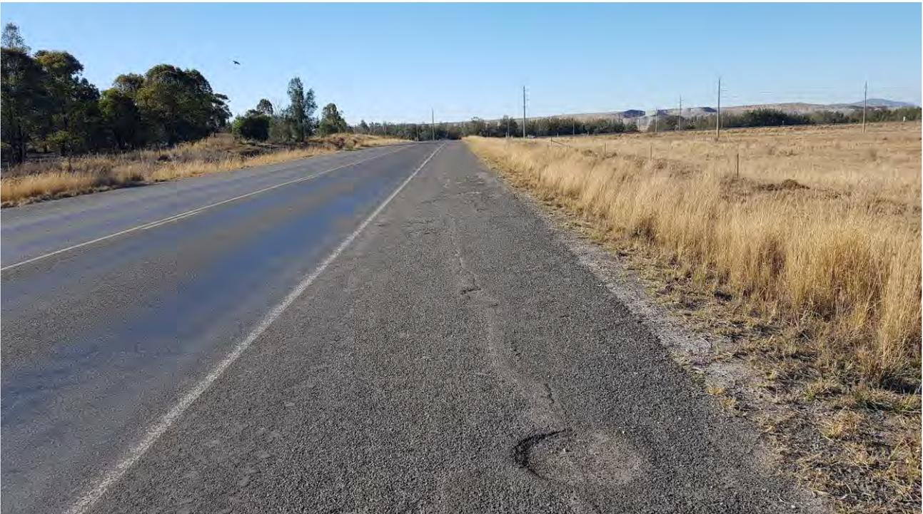
**Figure 9 - Looking North-East, cracking in shoulder with small potholes developing**
