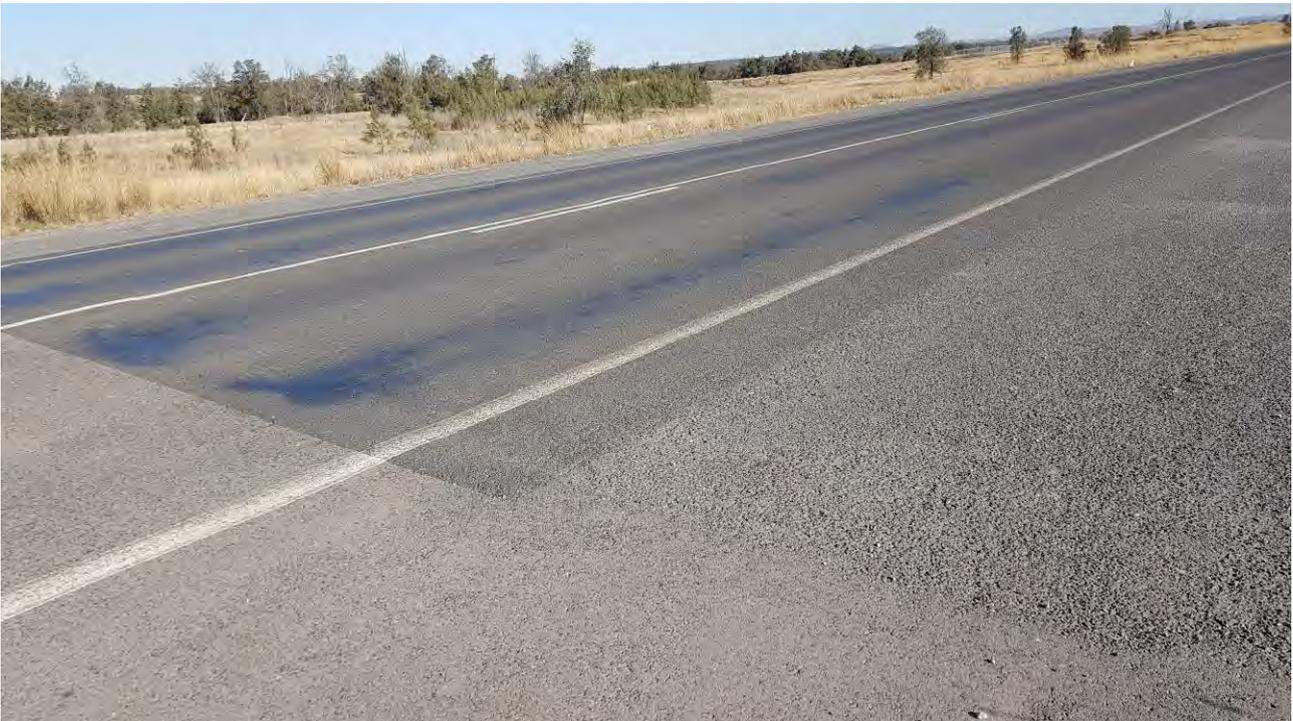
**Figure 21 - Looking South, joint of 2 pavements, no defects visible**
