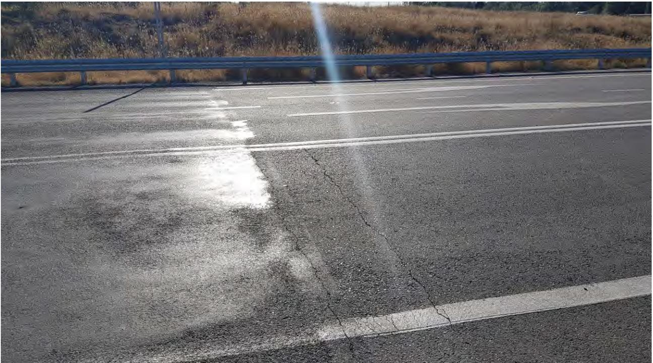
Figure 13 - Looking North-West, joint of 2 pavements, small cracking at joint and lead up to joint, one lane wide
