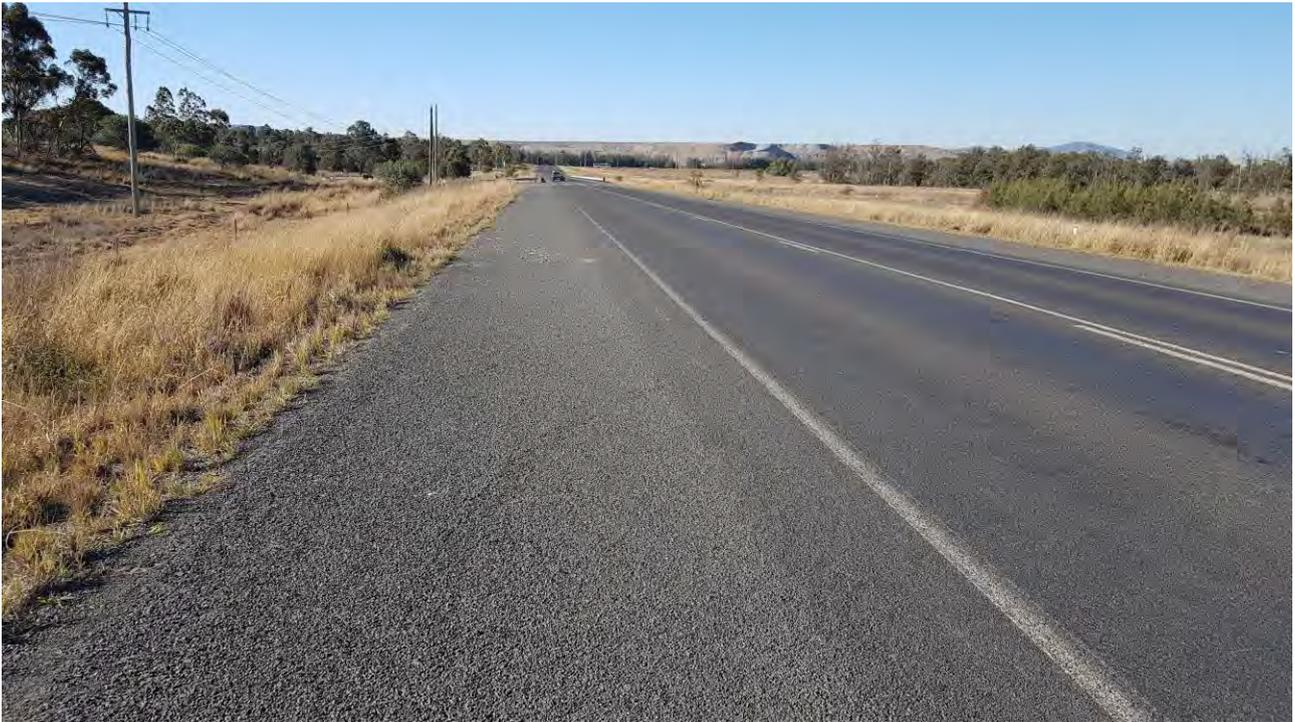
**Figure 22 - Looking North-East, no defects in laneway, minor wear in shoulder**
