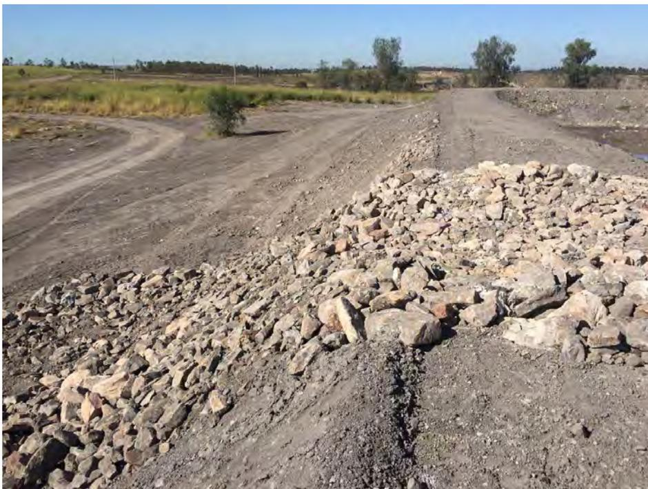
Photo 2 Rock lined overflow section on the eastern wall of the detention basin
