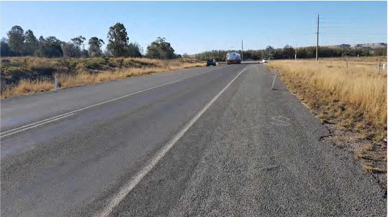
Figure 10 – Looking North-East, small depression in laneway where wheels travel, uneven shoulder
