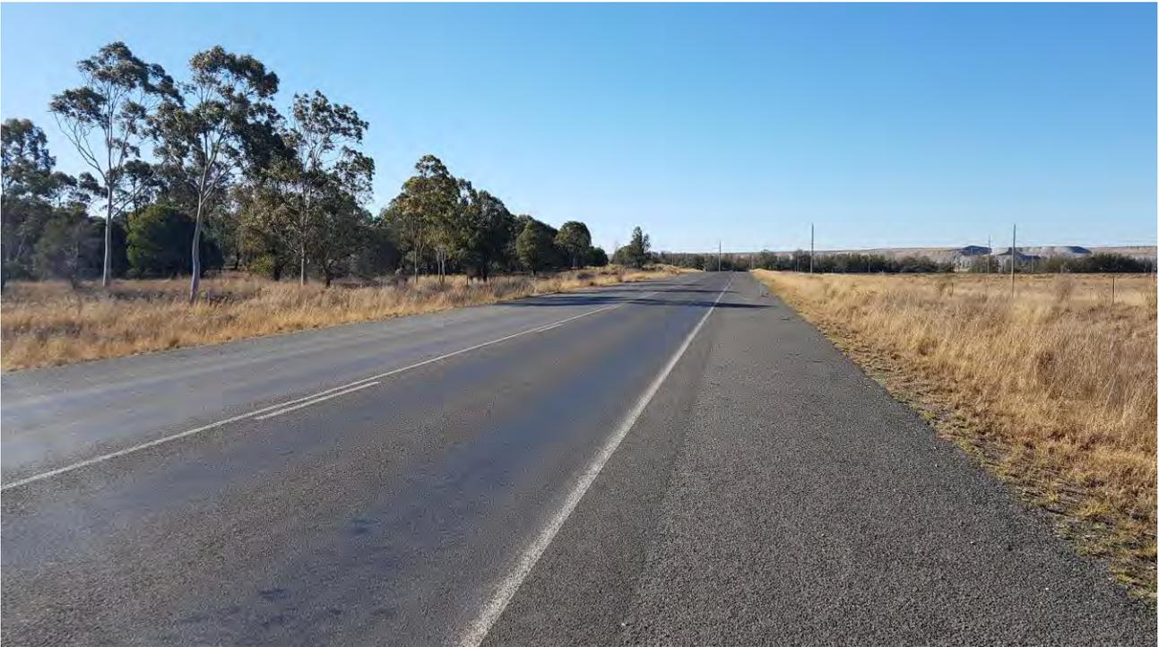
**Figure 8 - Looking North-East, no defects in laneway, minor wear in shoulder**
