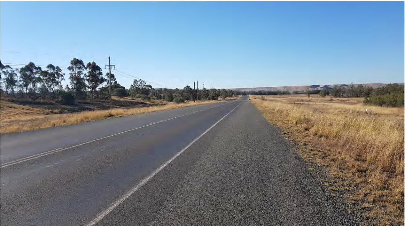
**Figure 3 - Looking North-East, no visible defects in laneway, minor wear in shoulder**
