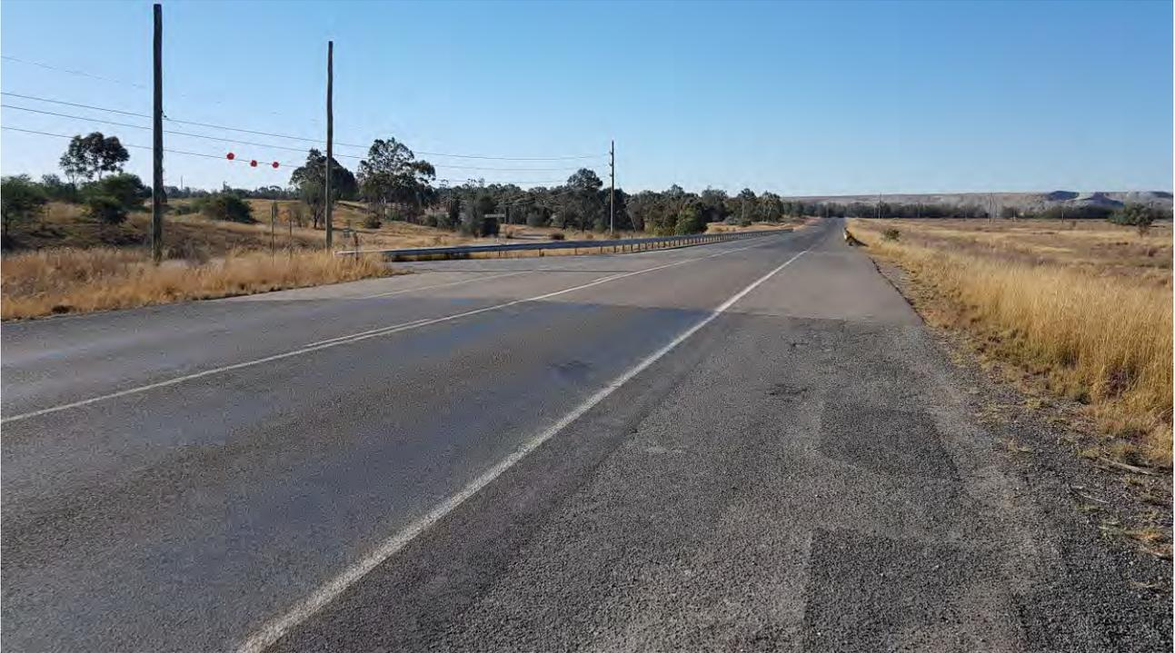
Figure 4 - Looking North-East, connection of 2 pavements, defects in shoulder and patchwork
