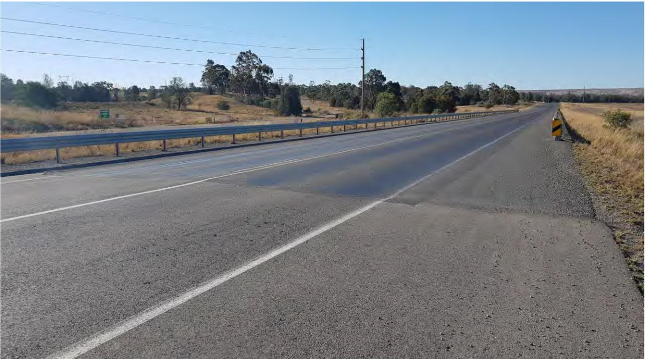
Figure 5 - Looking North-East, connection of 2 pavements, cracked area approximately 2m long by 1m wide
