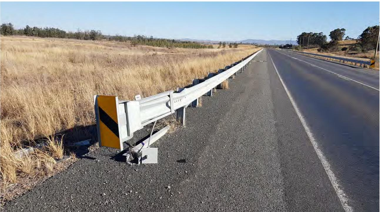
Figure 7 - Looking South, no defects in laneway, barrier damaged
