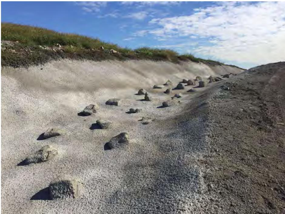
Photo 4 Looking up the shotcreted spillway channel
