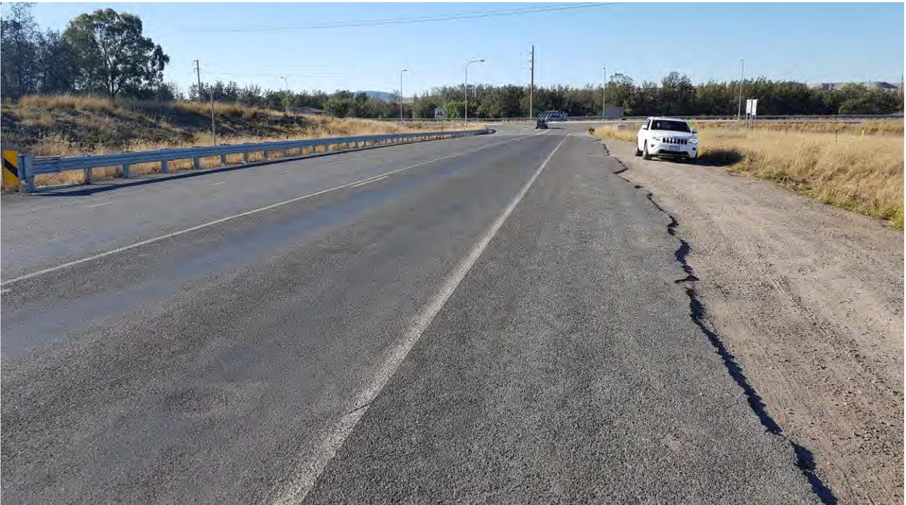
Figure 11 – Looking North-East, small depression in laneway where wheels travel, 40cm round pothole developing
