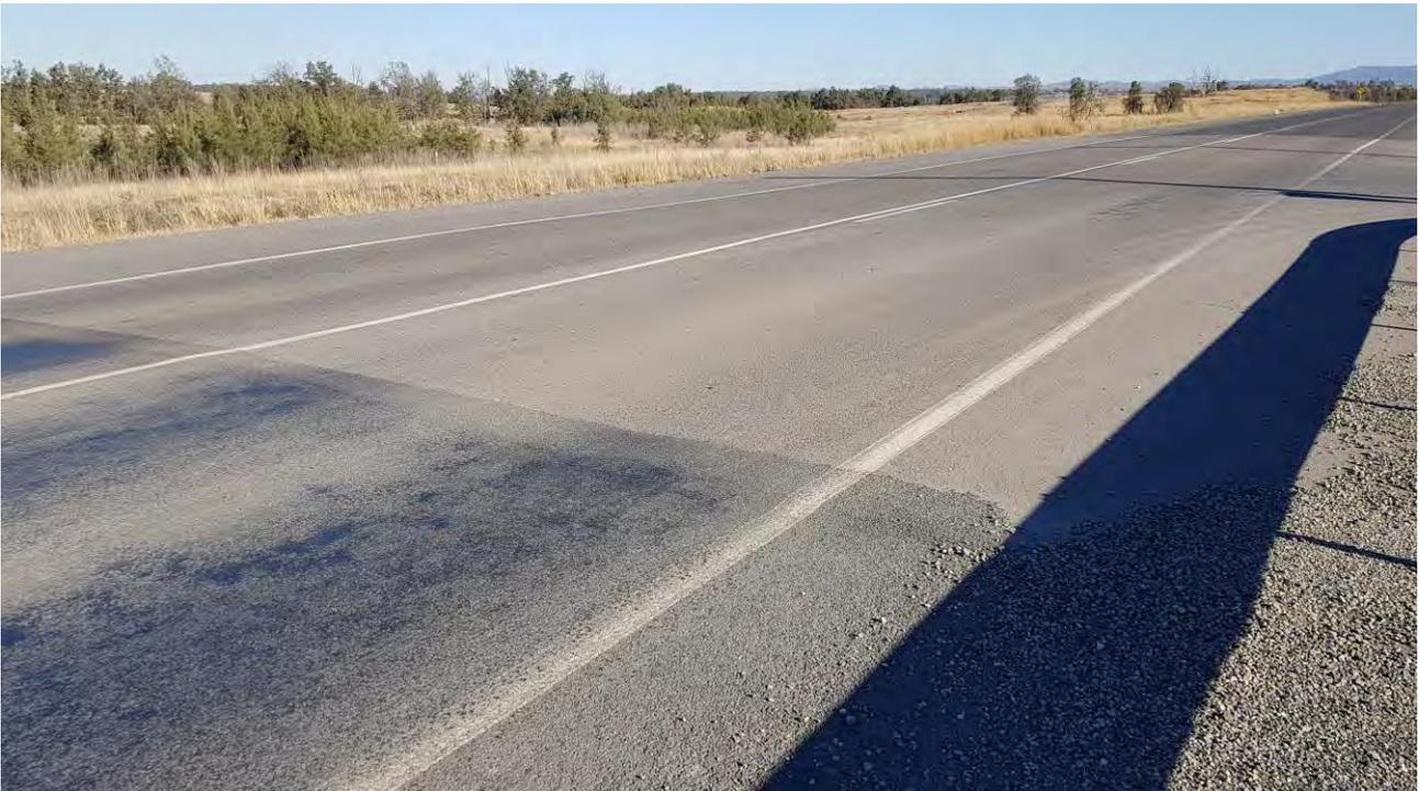
**Figure 19 - Looking South, Access to site, joint of 2 pavements, no visible defects**
