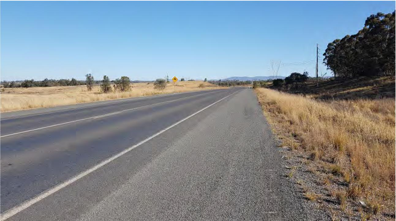
**Figure 2 - Looking South-West, no visible defects in laneway, minor wear in shoulder**
